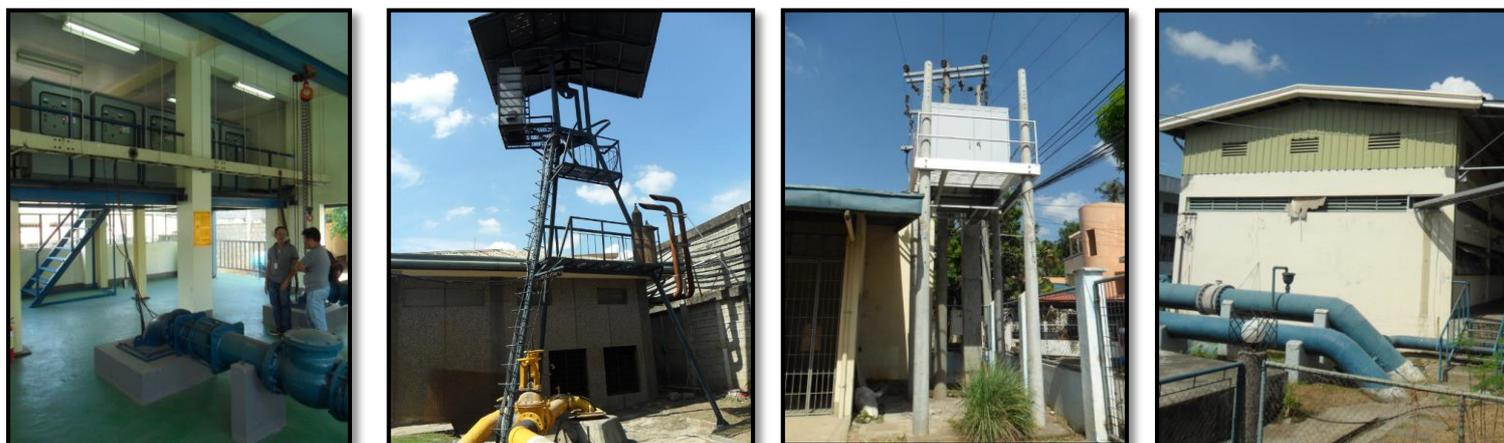
*From left to right: raised pump controllers and new submersible pumps; raised deep well controller; raised electric box; raised roof (green-coloured portion) on their pump house to accommodate raised controllers within. Source: Author's own (2015)*
